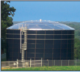
Municipal Potable Water
